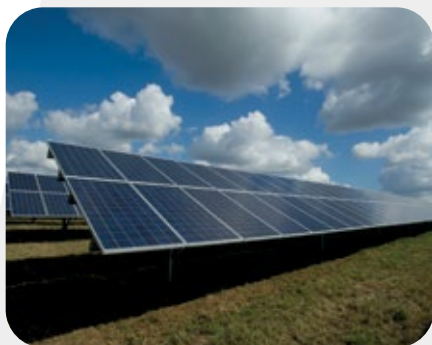
ENERGIE RINNOVABILI RENEWABLE ENERGY
