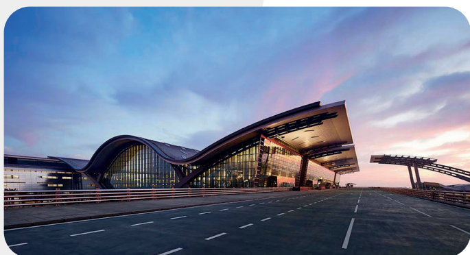
NEW DOHA INTERNATIONAL AIRPORT
