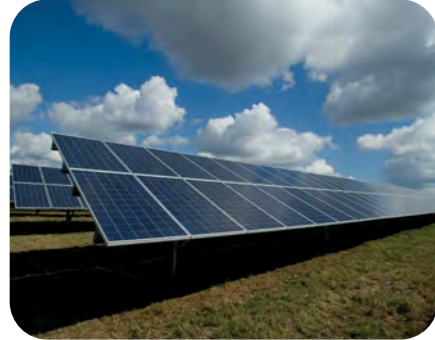
ENERGIE RINNOVABILI RENEWABLE ENERGY
